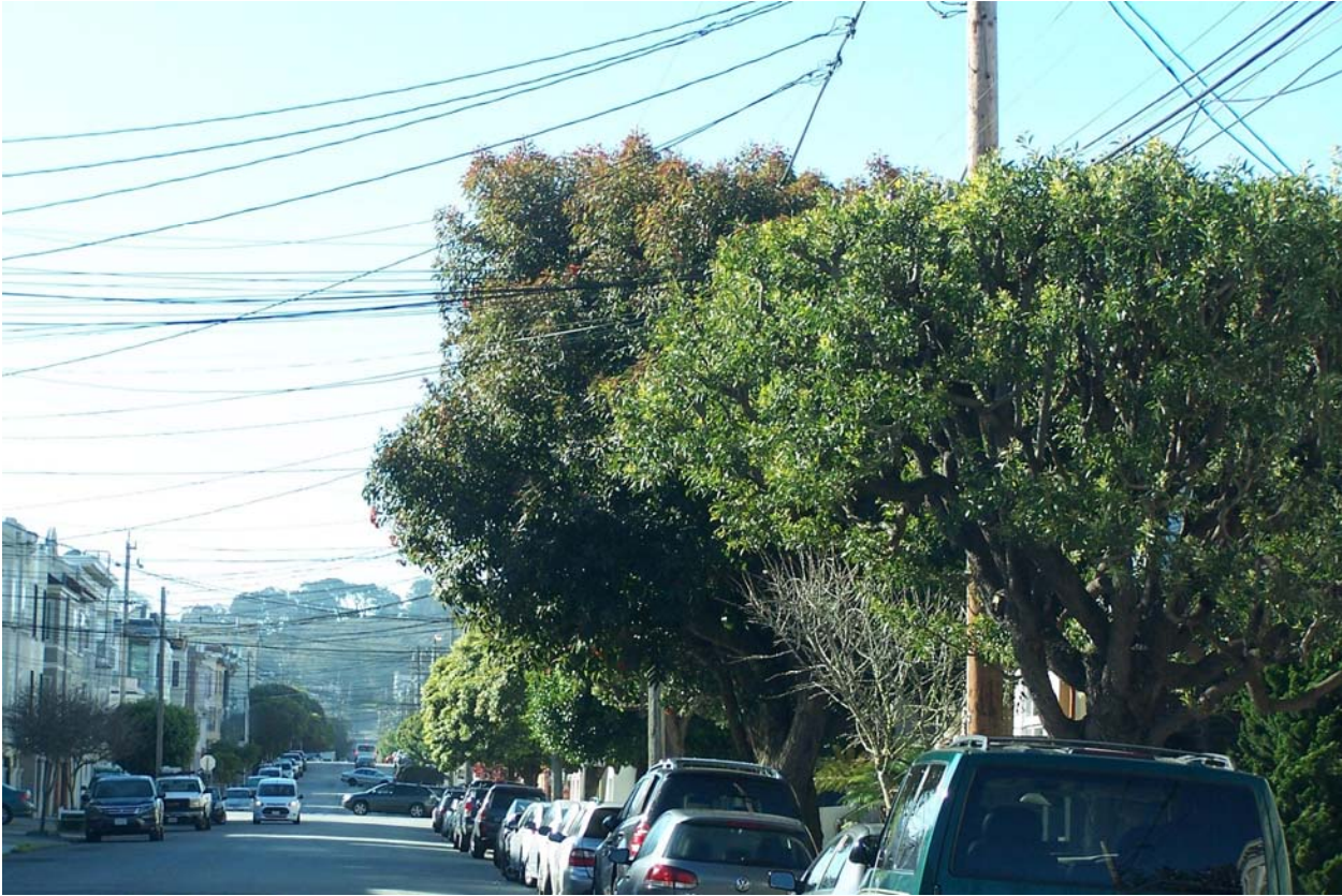
Figure 4: Tree Trimming Required on Richmond Pole Line
