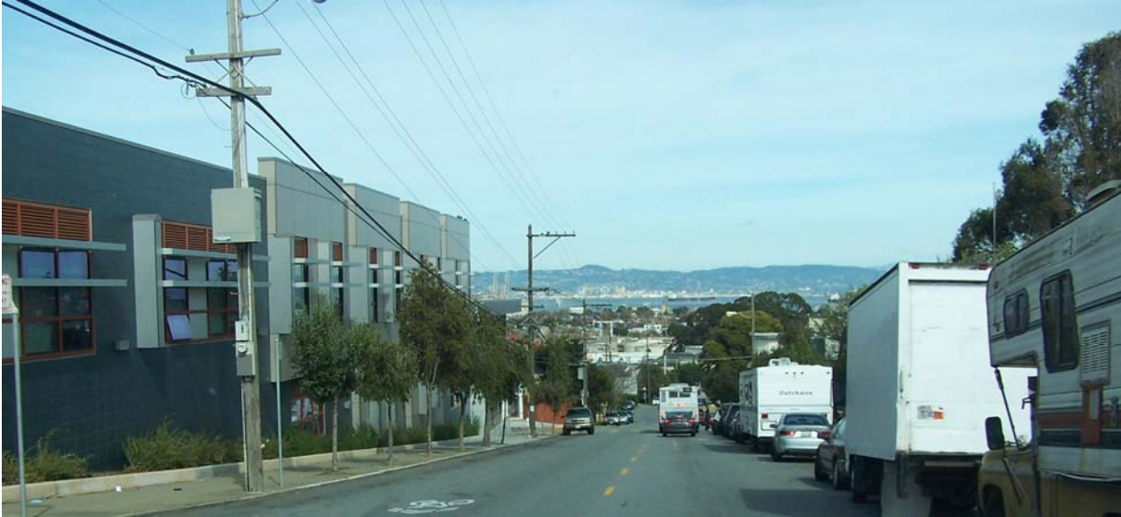
Figure 5: Clean Pole Line in Silver Terrace
