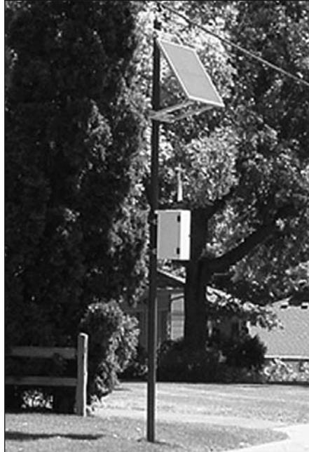
**A solar-powered wireless access point on a newly installed pole.**
