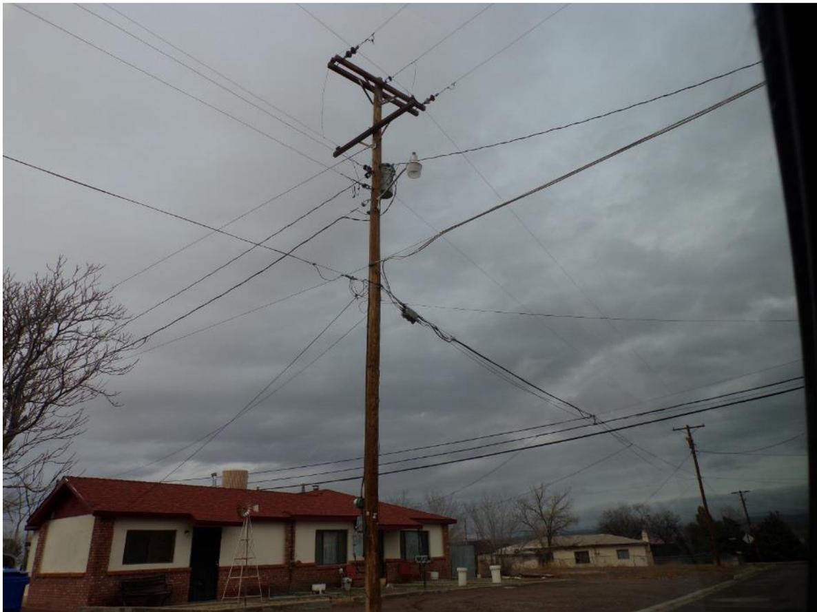
Near Espanola, we identified copper for DSL and dial-up on the poles, and middle-mile or backbone fiber underground (Figure 20).
