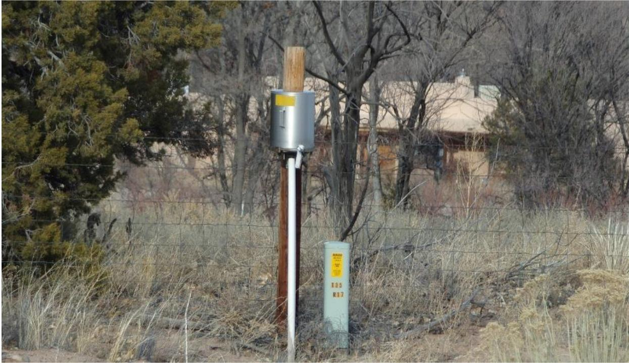
Near Deming, we identified the transition point from fiber to copper service (Figure 17). Copper lines only support DSL and dial-up; the fiber is for backbone and middle mile services only.
