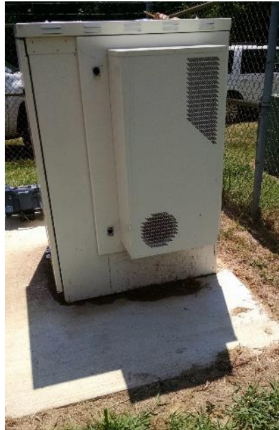
Figure 17: Fiber Distribution Cabinet
