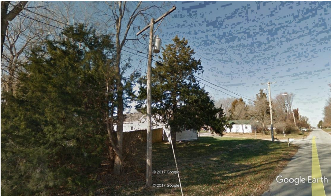
Figure 11: Congested Pole Line where Make-Ready will be Required
