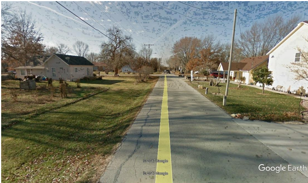
Figure 12: Example of Low Make-Ready Pole Lines
