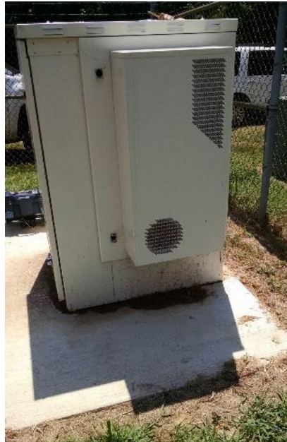
Figure 9: Fiber Distribution Cabinet
