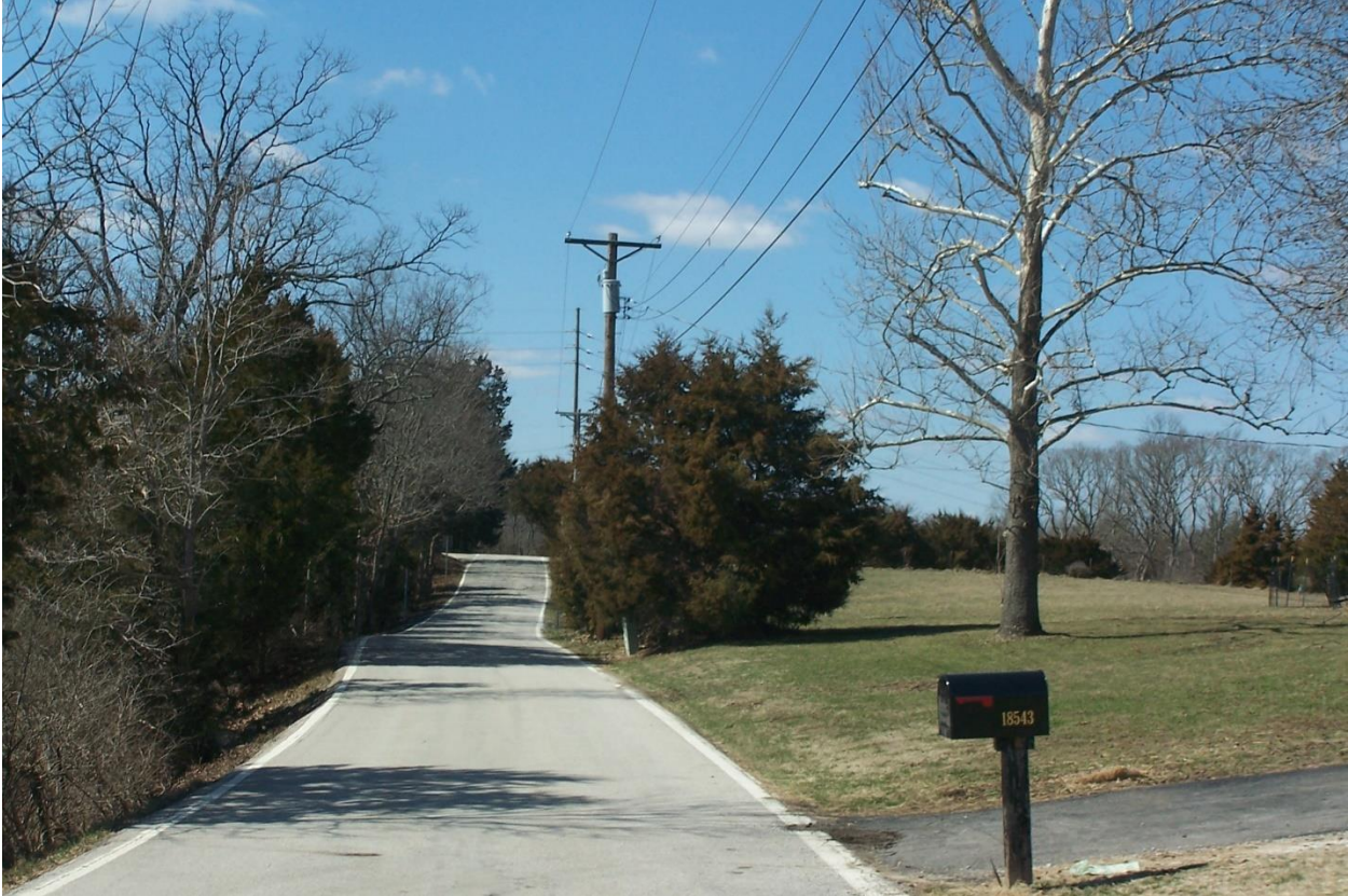
Figure 2: Utility Pole Line Showing where Tree Trimming is Needed
