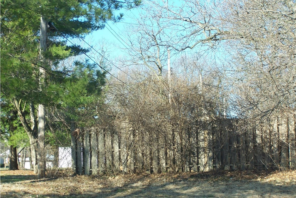
Figure 3: Congested Pole where Make-Ready will be Required
