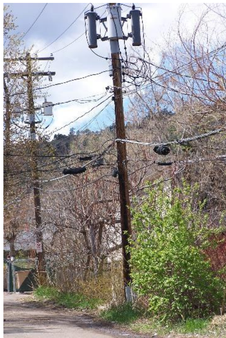
Figure 7: Make Ready Required on a Utility Pole
