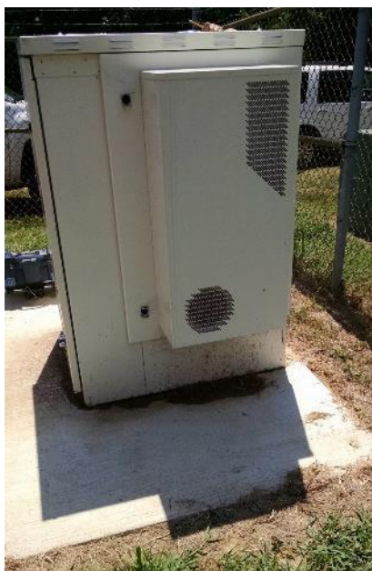
Figure 11: Fiber Distribution Cabinet
