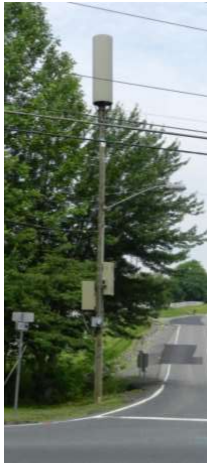
Figure 2 – Multifrequency DAS Structure with Multiple DAS Antennas
