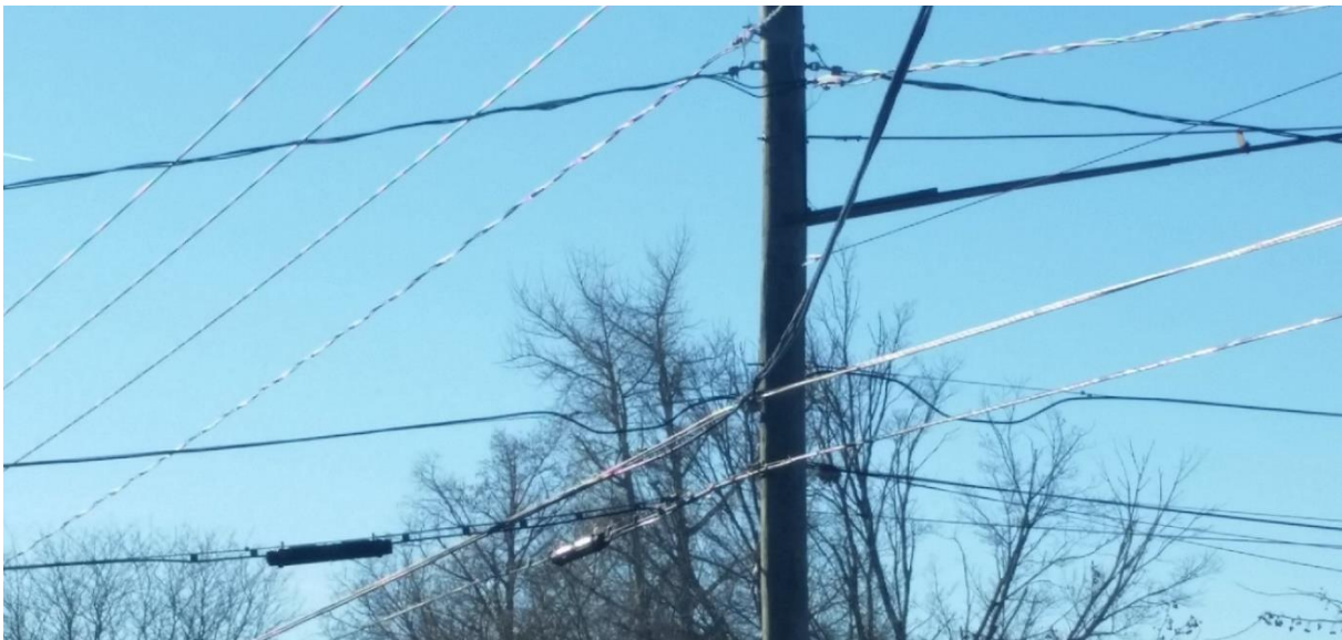
Figure 12: Congested Utility Pole in Sharon with Boxing on Both Sides of Pole
