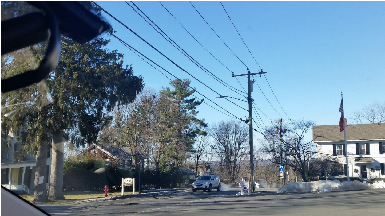
Figure 10: Sharon Hospital – Lighttower Cable and Splice Enclosure
