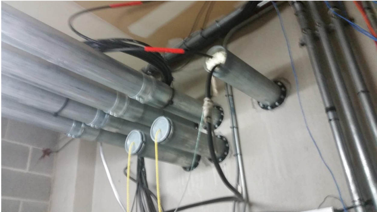
Figure 11: Geer Village – Self-Installed Conduit from Building to Street
