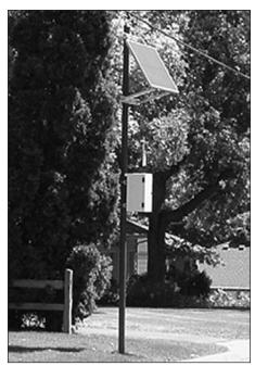
A solar-powered wireless access point on a newly installed pole.
